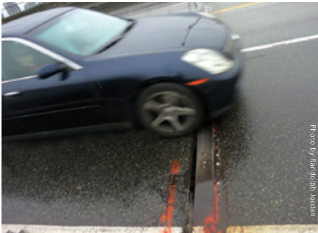
Fig. 1. (Left) Archival photo of Vancouver's Burrard Bridge, 1936. Fig. 2. (Above) Pothole atop of the southwest concrete pillar
